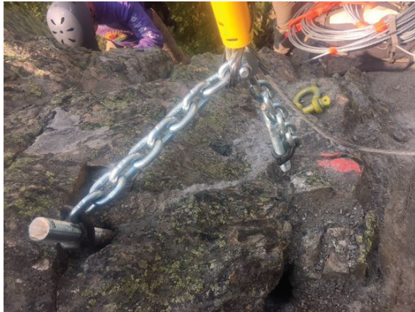
Figure 3: all-thread rods drilled and grouted into rock with guy wire
